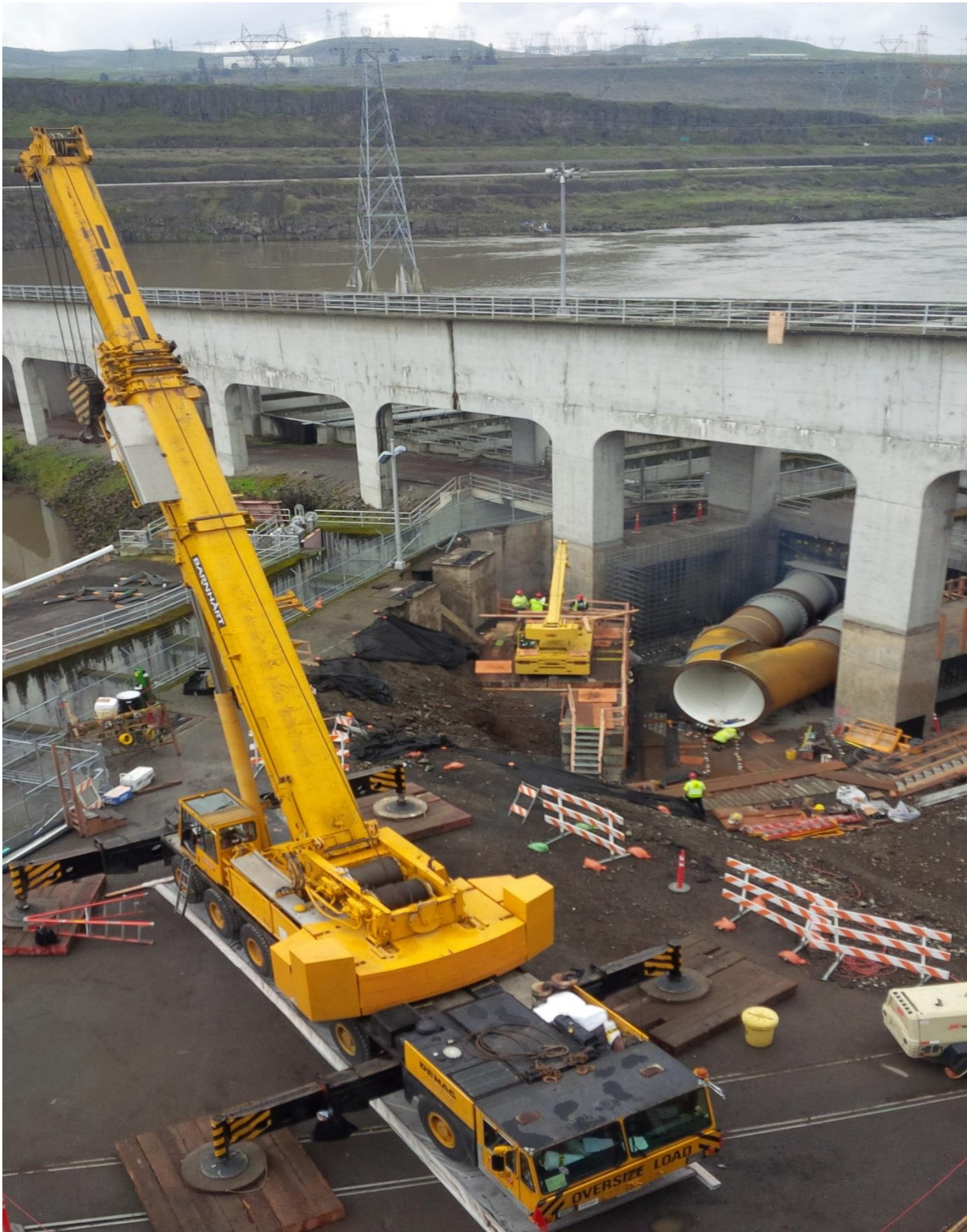
Bigger crane for bigger pipe.
